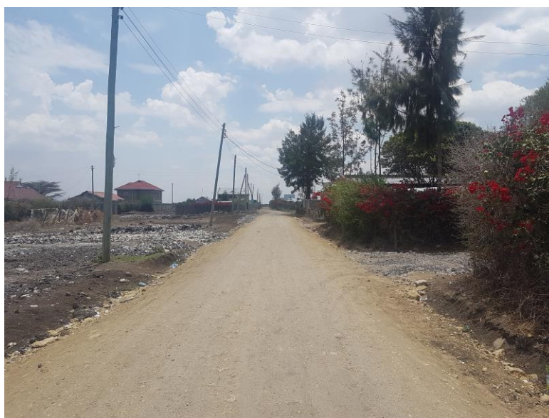
Photo of current site showing access road to be upgraded
