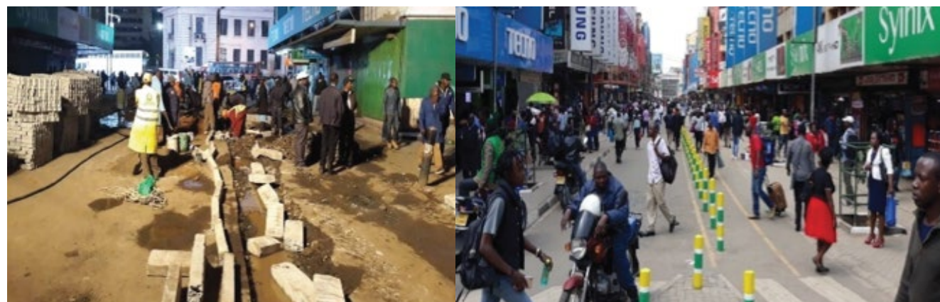
Luthuli Avenue before and after regeneration
